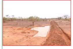
In the Rasko hedgerow perimeter, development work continued with the digging of trenches and infiltration ponds. Some ponds are already full following the first rains in June. In the coming days, we will begin installing the fence.
