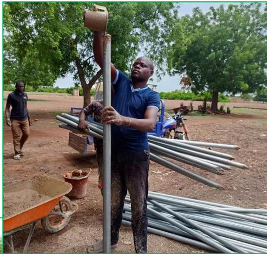
This year, reinforced concrete posts were used as boundary supports, replacing the wooden posts. The reinforced concrete stakes are made by pouring concrete into round tubes; these tubes are first cut to a length of about 2 meters, and then one end is sharpened. These stakes are very sturdy; over 2,800 were made by our technicians. Fences were erected to protect the newly planted trees.
