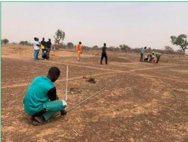
The development of the Mambogo bulli was one of CAF's main activities. After several topographical studies, the development work began with the digging of a double waterproof trench to serve as the foundation for the bulli's dike, followed by the digging of the spillway to drain excess water in case the bulli becomes full, and finally the digging of a large pond in the center of the bulli to store as much water as possible.
